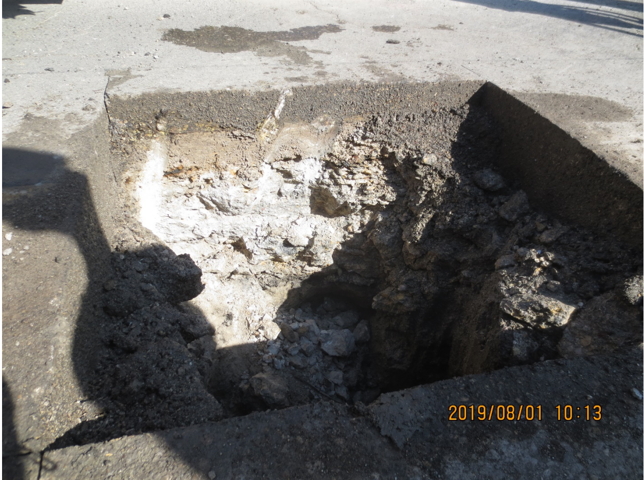
Figure 1 Streetcar Track Bedding below existing pavement (Station 2+360).
